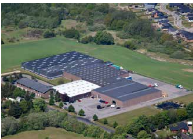
ERMAX A/S, Kolding, Denmark
