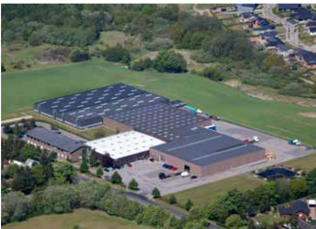
ERMAX A/S, Kolding, Denmark
